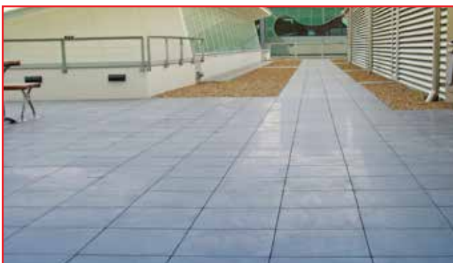
Chatswood Police Station, Australia
